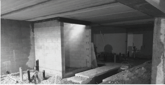
Elevator shaft as seen from the parish hall
